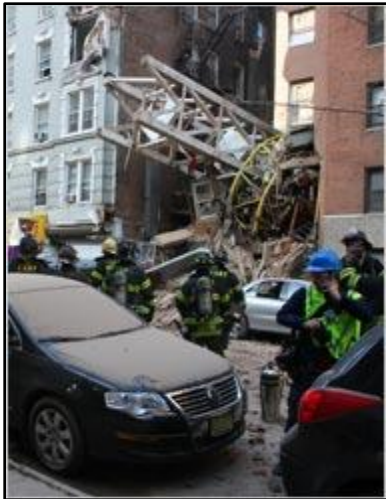
Emergency workers at the scene of a crane collapse at 51st Street and Second Avenue in Manhattan
